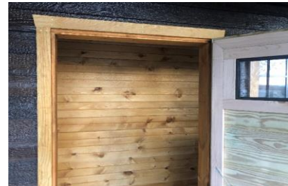
Interior Finish of Room Addition
