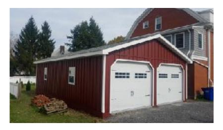
Same specs as vinyl garages except sidewalls with smooth LP Siding. 2x4 12" on center, Battens on exterior 12" on center. Includes paint.
