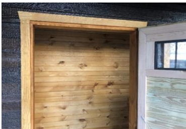
Finished Interior Pine T&G on walls and gable With Cathedral Ceiling
